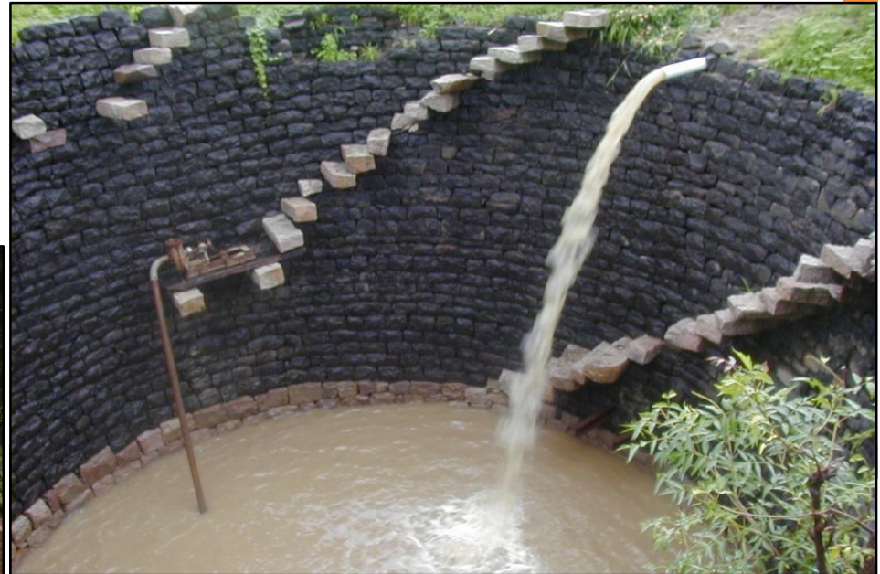
Low-cost mini percolation tank
